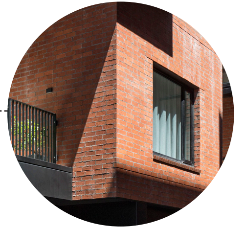
Red brick on timber framing. Mid-grey tone mortar. Red brick sill.
