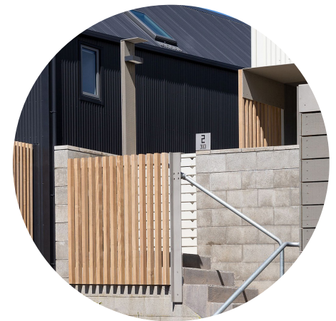
Solid fencing elements to entry. Planted for privacy. Communal 'letter box' in front of Unit 2.
